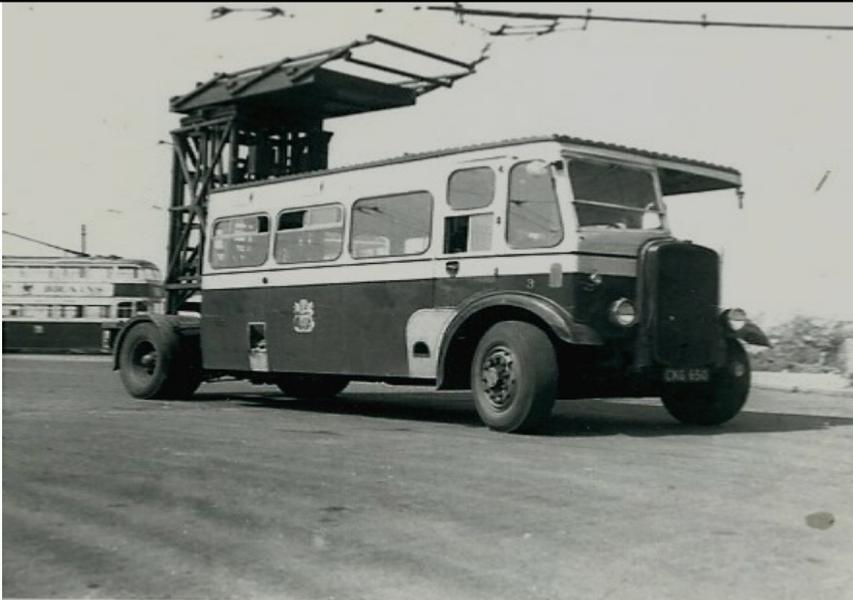
*This months front cover features one of the vital trolleybus ancilliary support vehicles. Tower wagon 3 started life in 1945 as motorbus 83, and served until 1960. On withdrawal it was converted in 1961, and remained until near the end of trolleybus operation in 1969, then like most of the vehicles it supported was sold to Bill Ways Cardiff East Dock scrapyard, another interesting part of Cardiff Trolleybus that failed to survive.*
